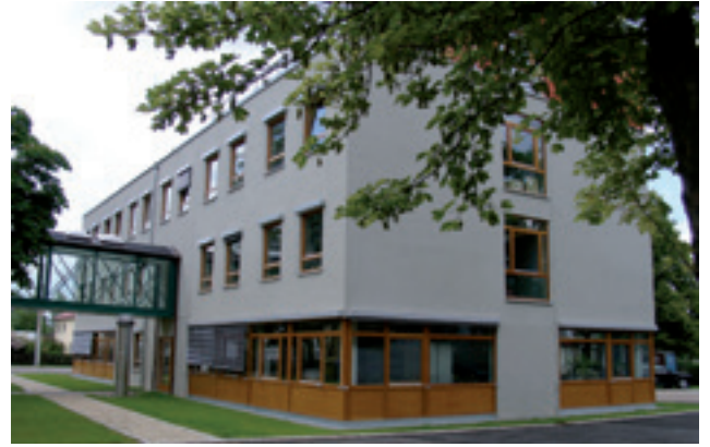
Building: Leipzig-Neukiritsch / Saxony (Newly constructed timber-framed building with UdiFRONT ® 60 mm)
