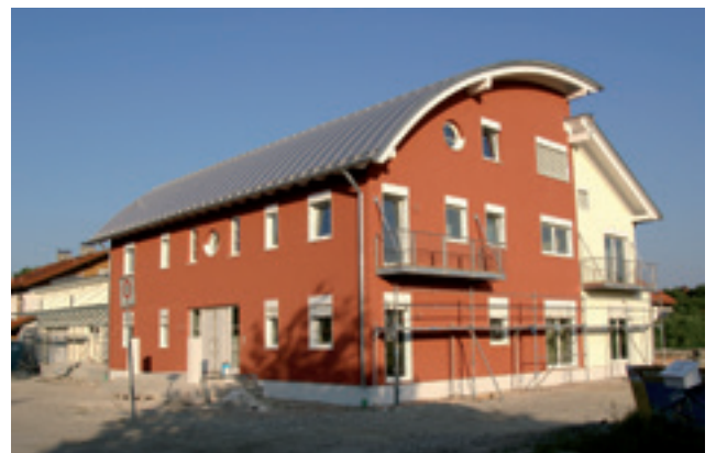
Building: BAUFRTZ Munich-Eichenau / Bavaria (Solid timber with timber-frame combination and UdiFRONT ® 60 mm)
