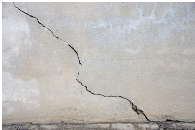
Cracks in the substrate
